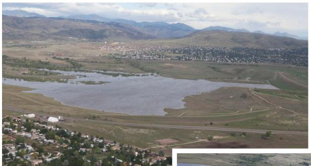
Bear Creek Reservoir near its peak elevation of 5607.8 ft, almost 50 ft into the Flood Control Zone, photo taken September 23, 2013
